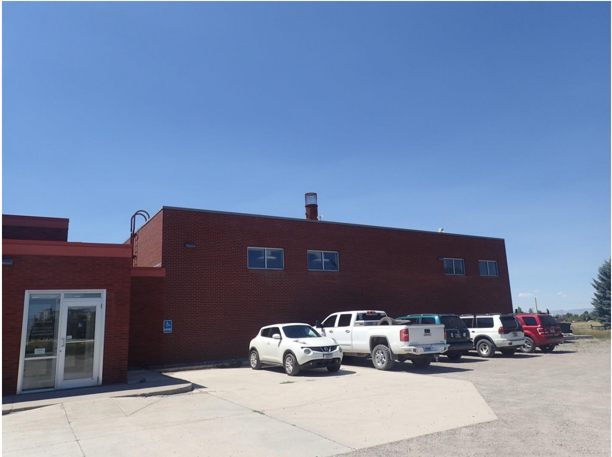
Figure 3. Incinerator Stack (Not Operating)
