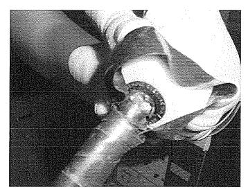
**Standard:** ARM 24.30.102; 29 CFR 1910.305(g)(1)(iv)(C). Unless specifically permitted otherwise in paragraph (g)(1)(ii) of this section, flexible cords and cables may not be used where run through doorways, windows, or similar openings.
